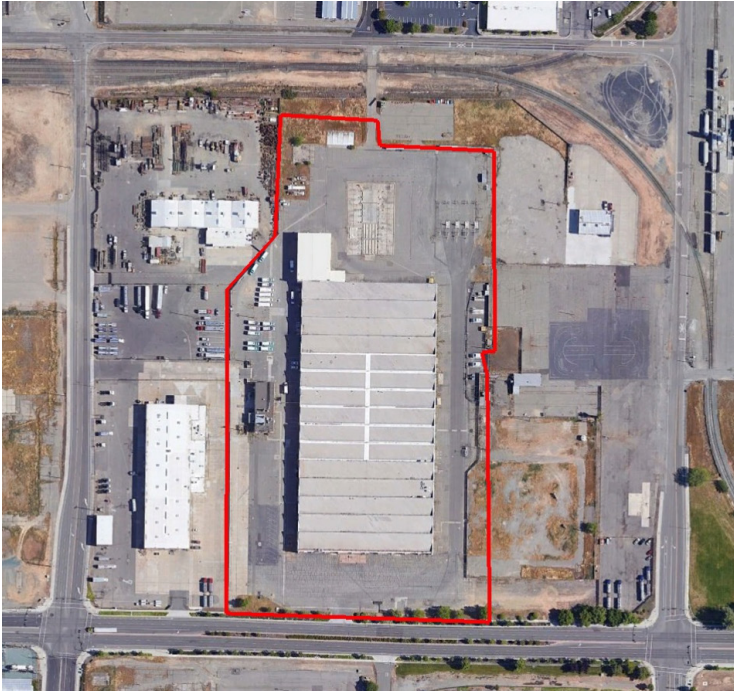
Figure 4-4 McClellan Garage - Existing Conditions | Source: WSP
